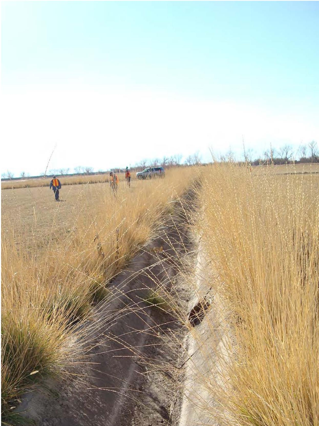
**Figure 4-3.** Example of a concrete-lined ditch in the Project Area.
